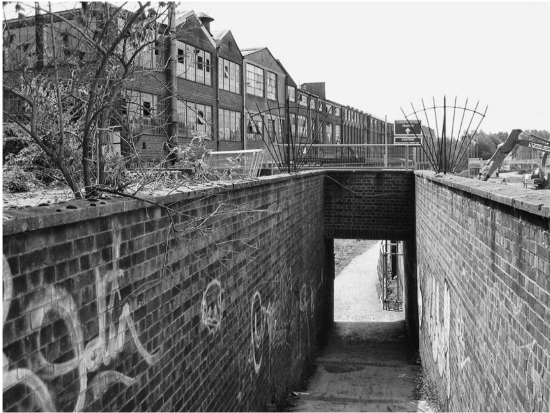
Figure 7.5 Derelict land and accompanying graffiti and litter can lead to misuse and perceptions of insecurity, deterring users.
