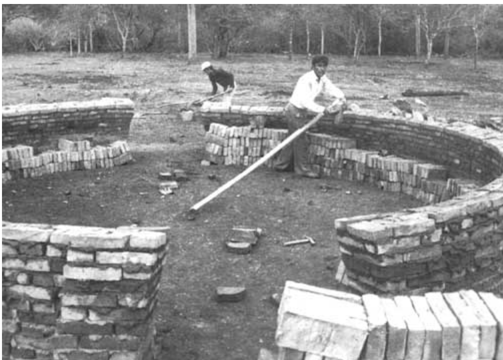
Photo. 14. Building a half orange brick kiln. Note the wooden radius rod, the way the bricks are laid and the double layer of bricks over portion of the wall to reinforce the shell of the kiln. Argentina. Photo. J. Bim.
