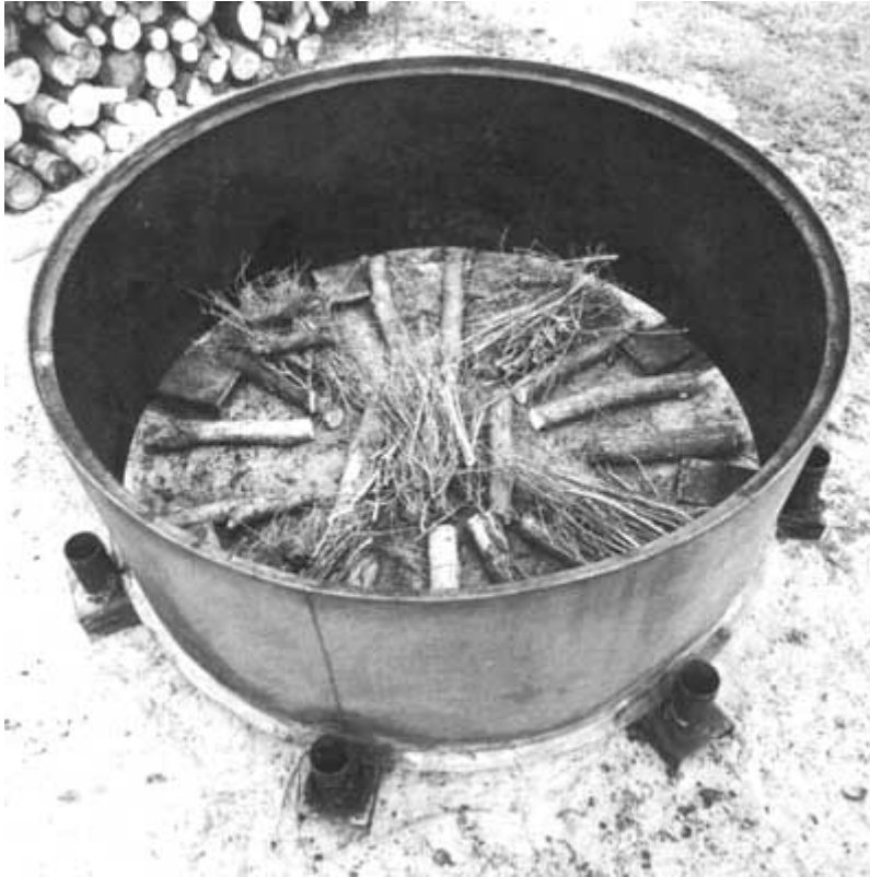
Photo. 30. Inflammable waste is placed between the stringers to provide four lighting points. Photo. TPI
