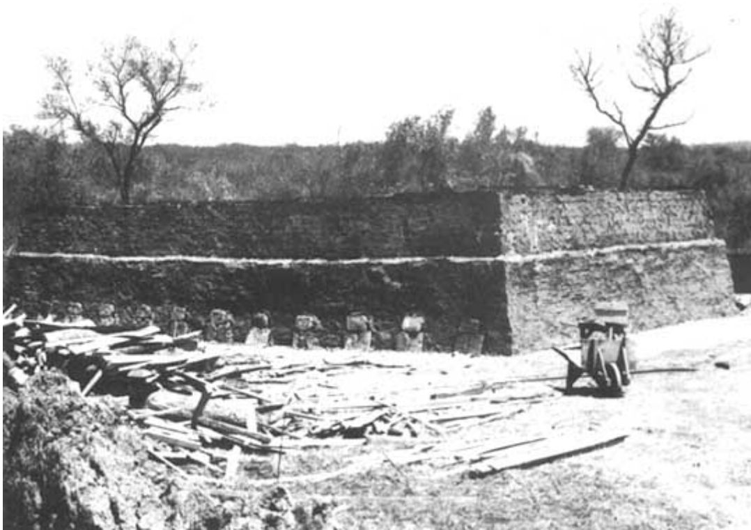
Photo. 20. Brickmaking using hand methods and fired in a pile with flues using wood fuel. Embarcación, Argentina. Photo. H. Booth.
