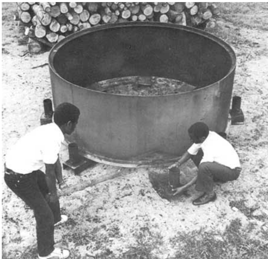
Photo. 28. Assembling of metallic kiln. Photo. TPI
