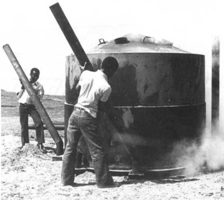
Photo. 33. Joints between the main sections of kiln are filled with sand or soil and smoke stack is placed into position. Photo. TPI
