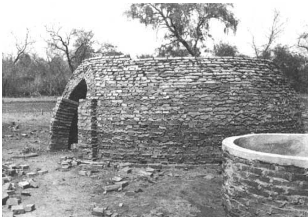
Photo. 17. Partly completed half orange kiln and completed water storage tank. Note cross bonding of brickwork in the double layer part of wall and way bricks are laid in the single layer section. Argentina. Photo J. Bim.
