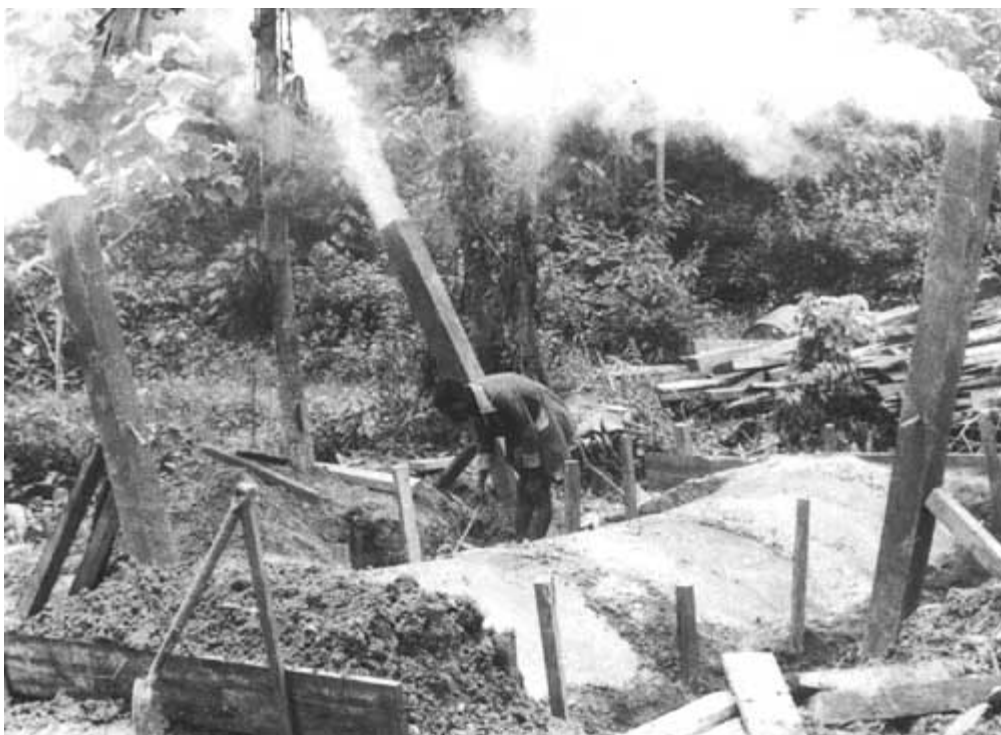
Photo. 7. Earth pit during burning. Note steel chimneys and cover used made of steel sheets sprung between stakes. Joints between sheets sealed with earth. Ghana. Photo. Lejeune.
