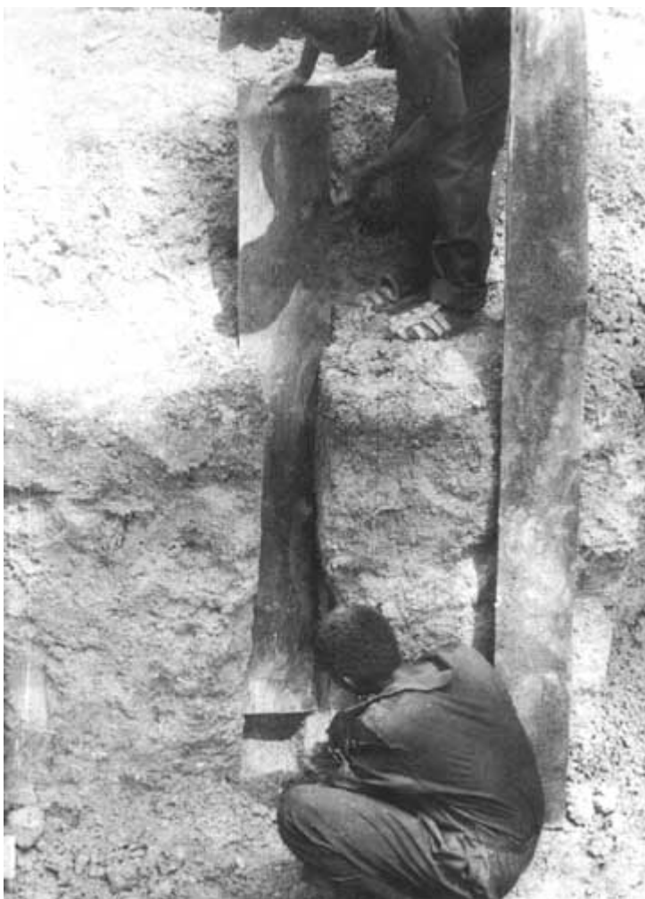
Photo 8. Vents for pit kilns can be timbered where soil is loose avoiding the need for steel. Ghana. Photo Lejeune.
