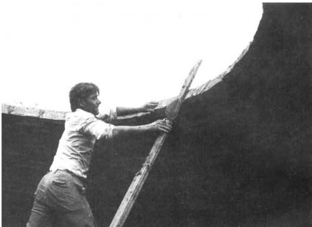
Photo. 16. Closing dome of a half orange kiln under construction. Note radius rod and orientation of bricks in dome. Argentina. Photo. J. Bim.
