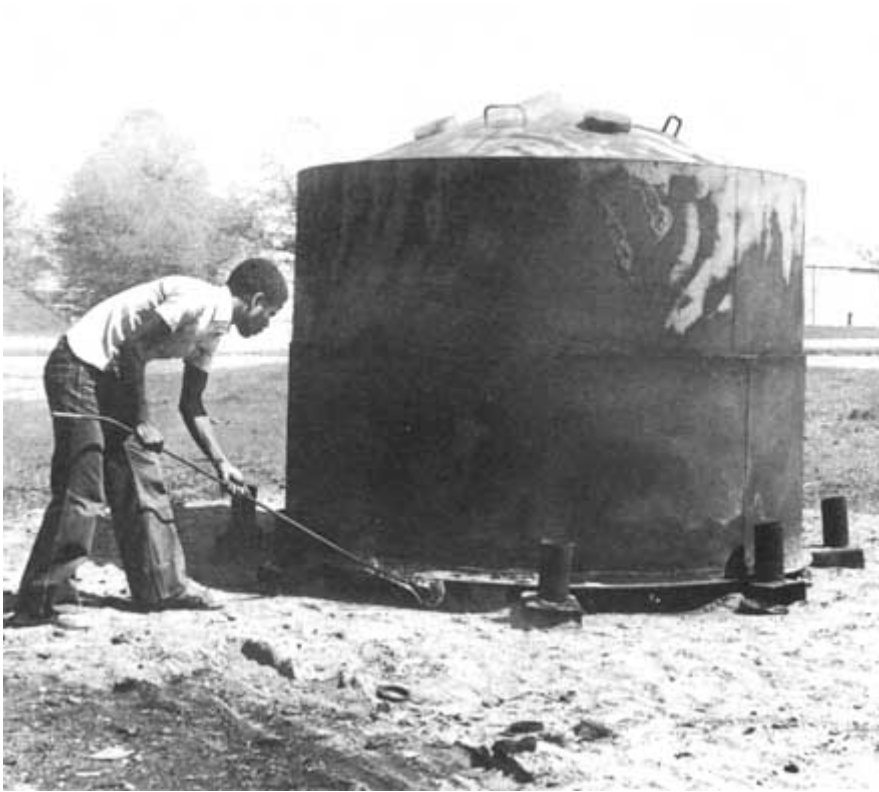
Photo. 32. Lighting points. Photo. TPI
