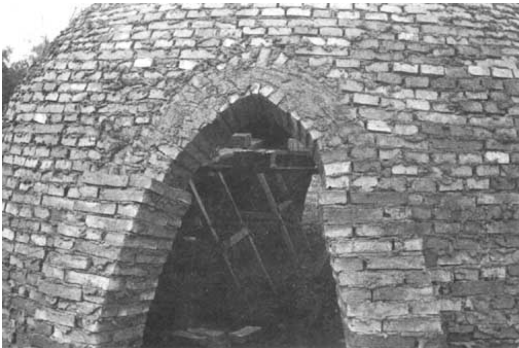
Photo 15. A half orange kiln just built. Note reinforced doorway to avoid damage to kiln during loading and unloading. Note way bricks in double skin wall around door are cross bonded compared with single layer wall seen in top right-hand corner. Argentina. Photo. J. Bim.
