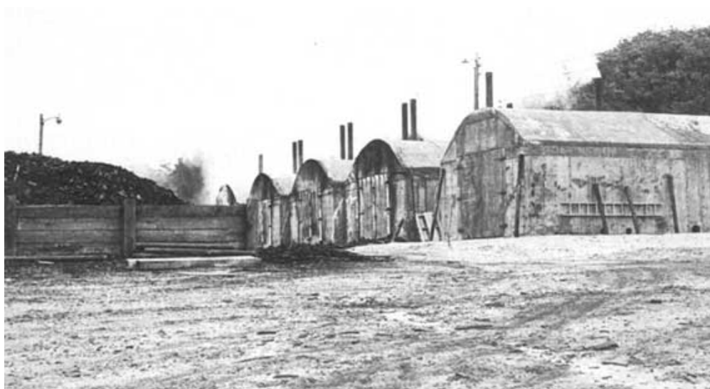
Photo. 13. Missouri Kilns made of reinforced concrete. Note steel doors, charcoal stockpile. Missouri, U.S.A. Photo A. Baker
