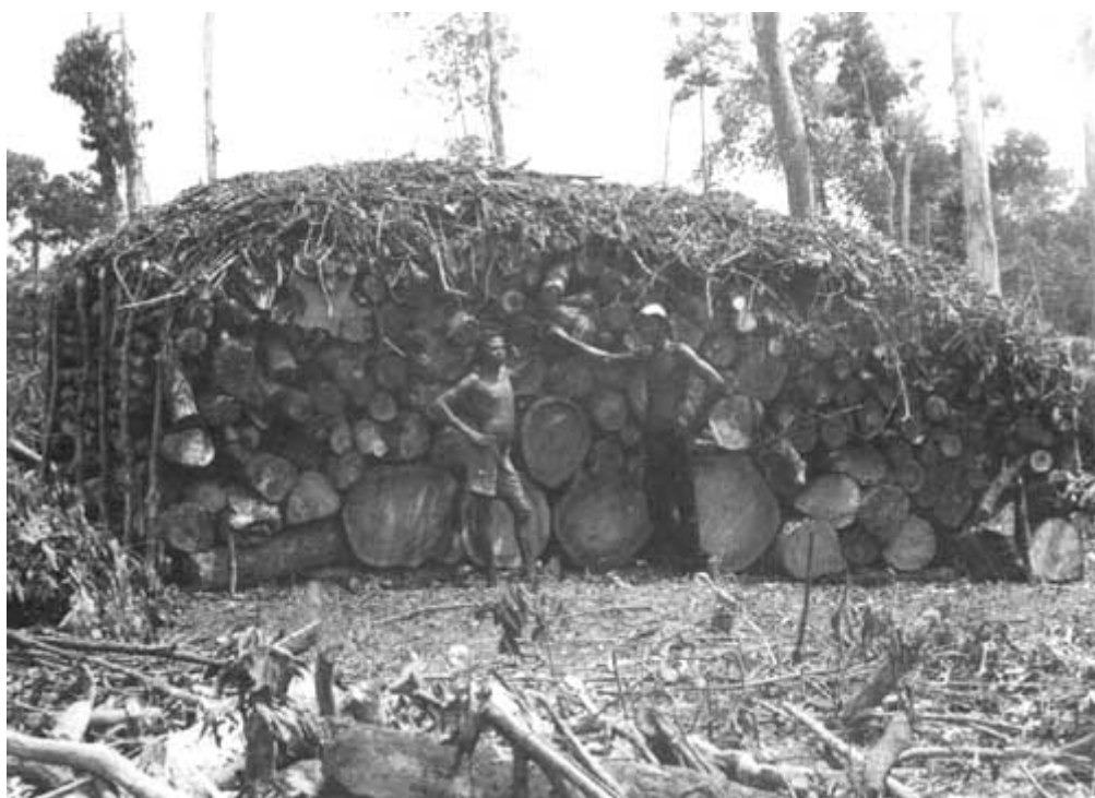
Photo. 11. Earth mound kiln during construction. Note large diameter wood placed at base of pile. Ghana. Photo Lejeune.
